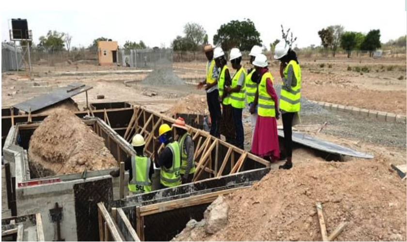
Training on casting foundations
