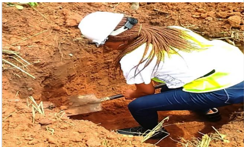
Training on excavation work for street light plinths
