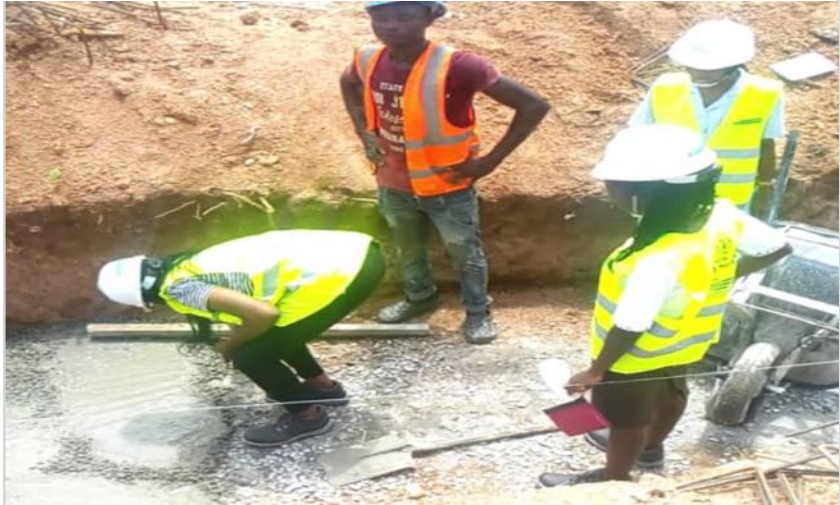
Training on retaining wall base
