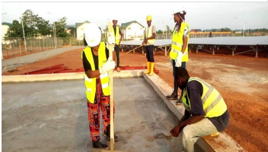
Training on PCC of BBR foundation works
