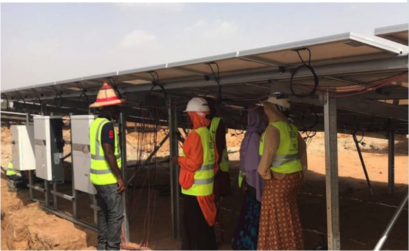
Training on DC cable tagging for the PV strings
