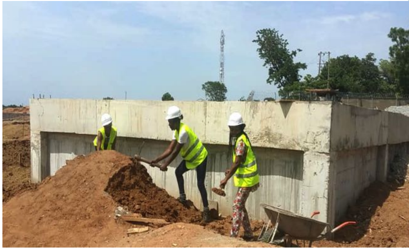
Training on backfilling of the completed equipment foundations
