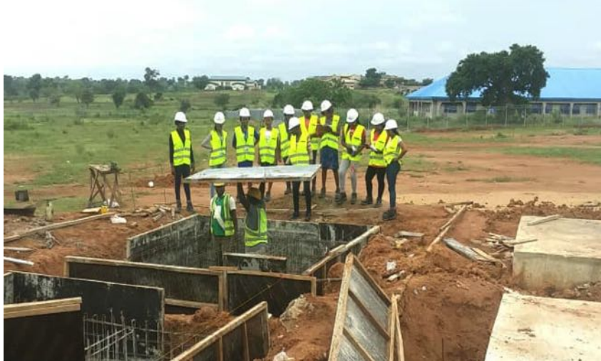
Training on the installation of transformer foundation plinth beam formwork
